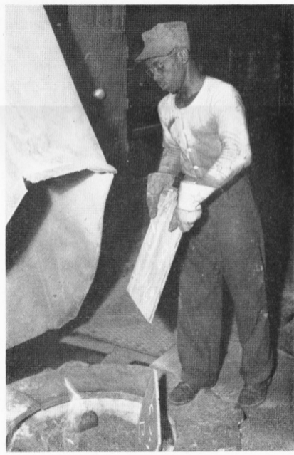
Leather-palmed, canvas back gauntlets have been found best suited for work in the Casting Shop. Edward Washington feeds a copper slab into an Ajax Electrical melting furnace.
